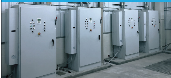
H 2 S corrosion resistant control panel cooling
