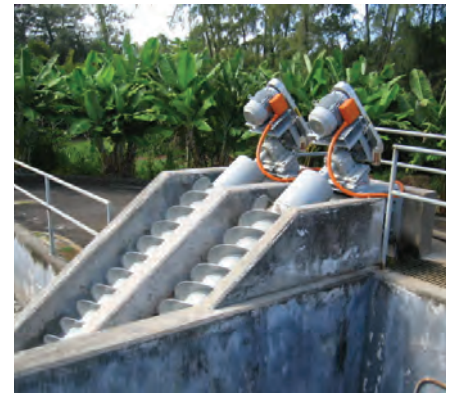
Non-clogging screw pumps from Lakeside have been installed at several locations in Hawaii.
