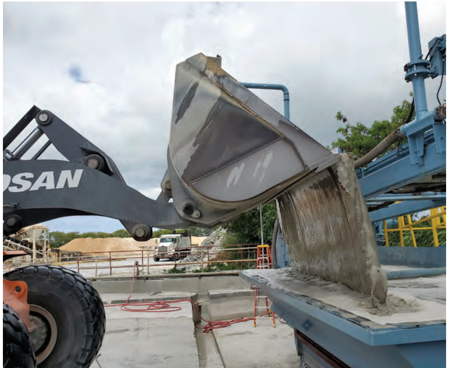
New washout systems offering potential savings and additional revenue to concrete producers.
