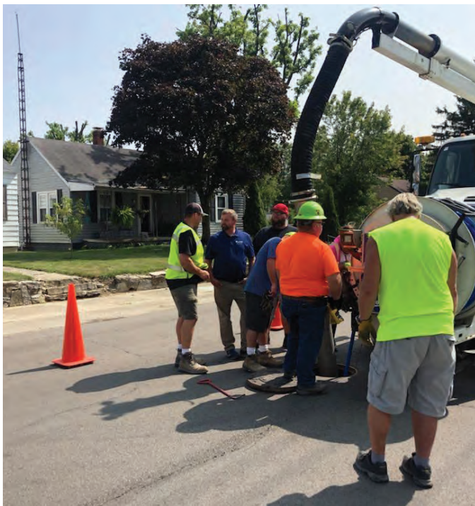
When the water flow confirms the pipe has been cleaned at the right speed, the maintenance crew can lower the pressure in the hose and come back through the pipe at the same speed.
