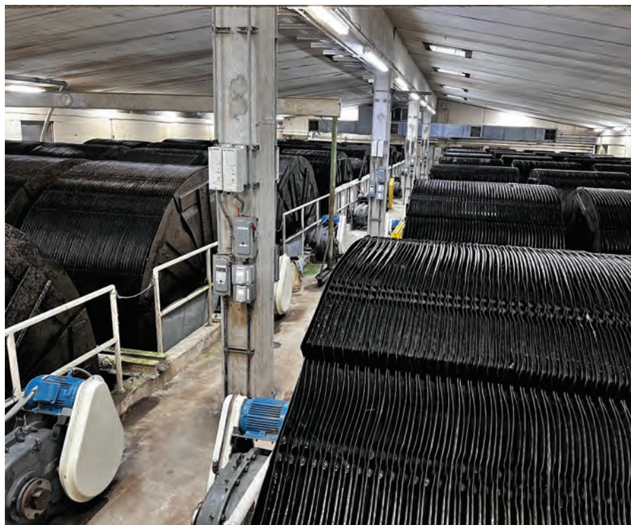
Rotating biological contractors used in secondary treatment process.
