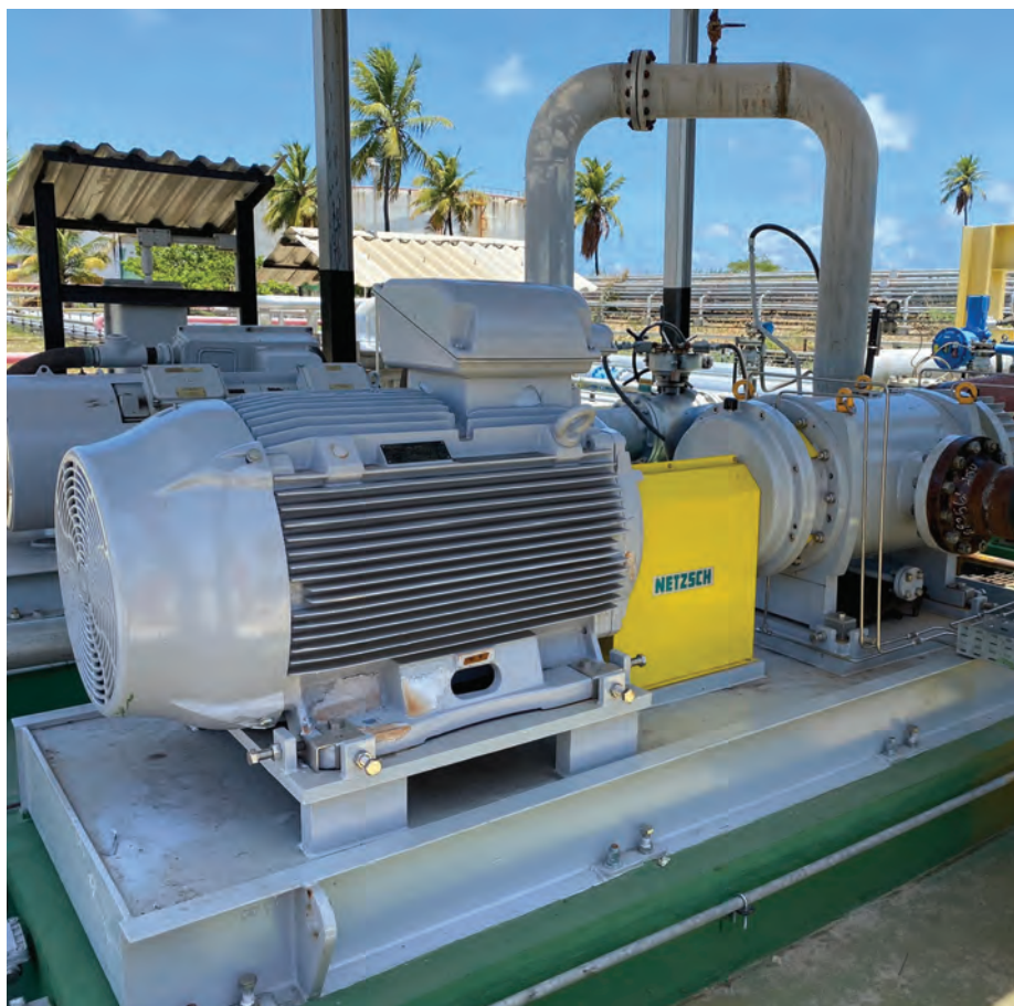
The overall energy costs were lowered significantly, in particular because the second existing centrifugal pump was also replaced with a 4NS after the successful test phase in February 2020.
