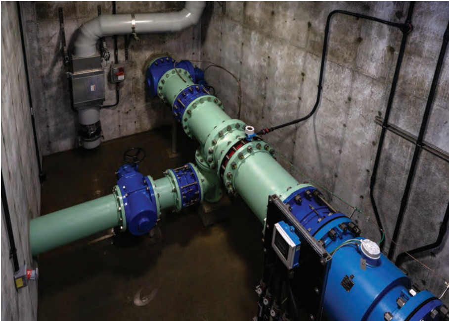
The new station includes four new pumps, process pipes and grinders.
