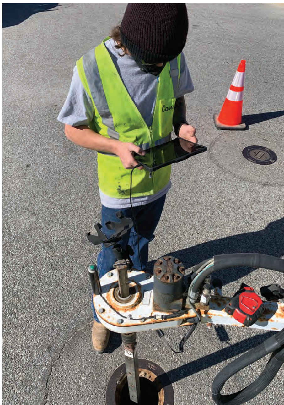
Sedaru and Wachs valve exercising machine work together to eliminate operator error.
