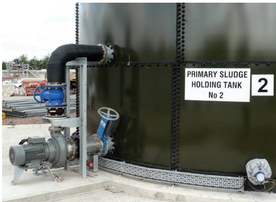
Similar to Landia's proven AirJet aeration system, JetMix is externally-mounted for easy servicing.
