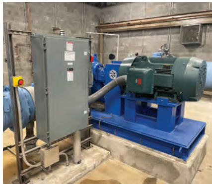
At both locations, sophisticated electrical systems support efficacy with each of the pumps paired with a high-efficiency variable frequency drive (VFD) which optimizes power usage and pump productivity.
