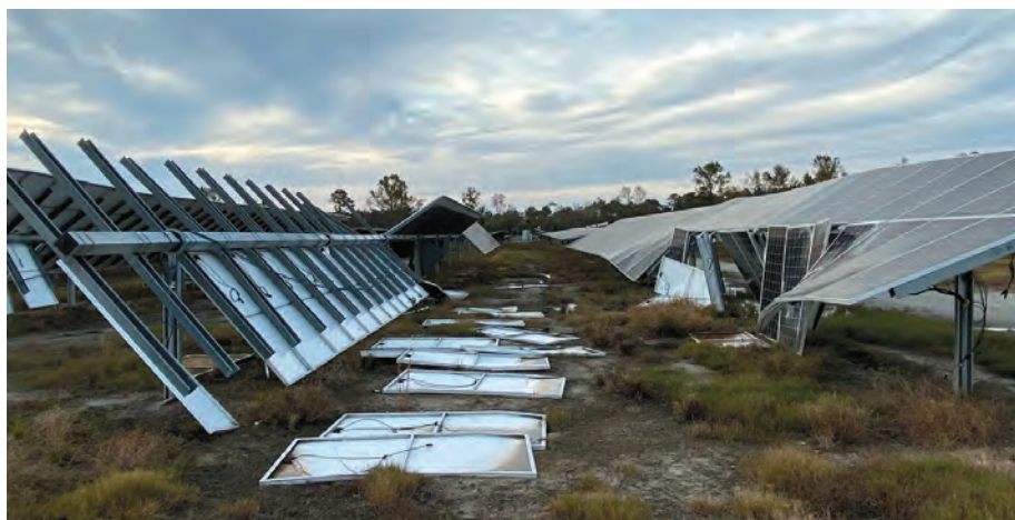
80 MPH winds damaged 15 percent of one site's trackers.
