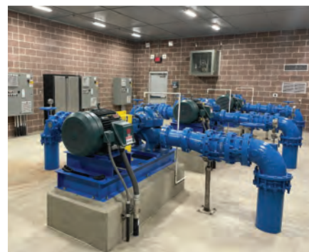
Three Xylem e-XC Double Suction Centrifugal pumps run on efficient drives at the Hartselle project. They operate as demand requires under several conditions, such as a baseline, minimum target water pressure of 60 pounds, and a full flow rate of 1,200 gallons per minute.
