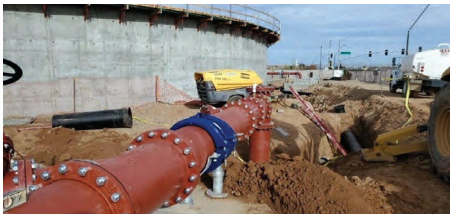
The HYMAX® Grip Large Diameter (LD) 16-inch restraint coupling installed at Queen Creek's new water storage facility.
