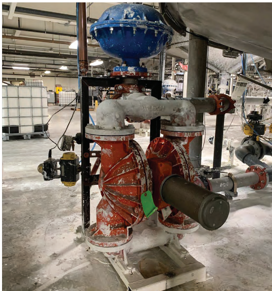
After seeing how Wilden Chem-Fuse IPDs can improve service life and pump performance, Dunn-Edwards will begin standardizing the use of Chem-Fuse diaphragms on all of the 3-inch Wilden AODD Pump models in use at its Phoenix, Arizona, manufacturing plant.
