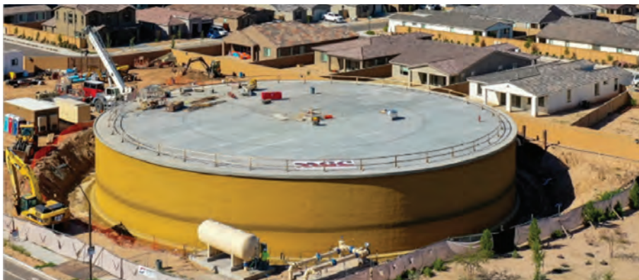
Queen Creek's new three-million-gallon pre-stressed concrete storage tank.
