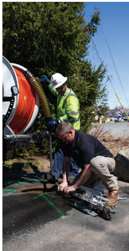
For safety in sewer pipe, open the upstream sewer manhole first, and this will allow the system to draw in fresh air.
