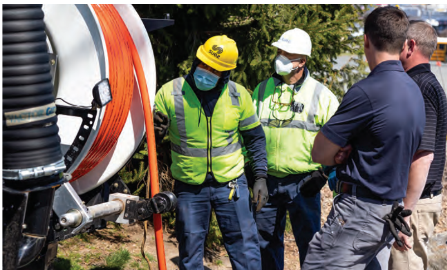
To prevent free spooling the nozzle up the line and losing control, use a nozzle skid and hold the nozzle back.
