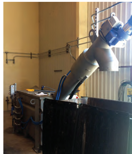
By capturing debris from the septage, damage to downstream equipment, such as clogging pumps, is prevented.
