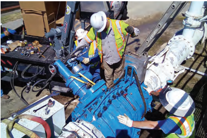
The EM machine milling a 120-degree slot across the top of Pipe #5.
