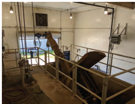
The Lakeside Screen is extremely effective in removing rags and plastics.
