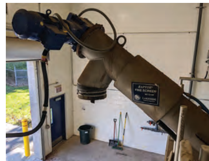
The rotating rake teeth of Lakeside's Raptor Fine Screen fully penetrate the cylindrical screen bars.
