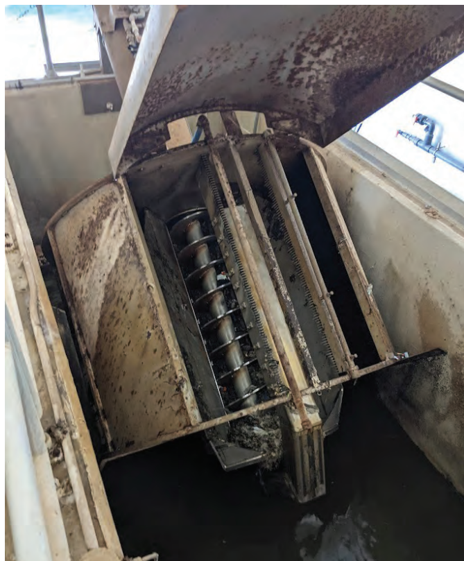
Angled installation and screen bars of varied heights increase removal efficiency and minimize head-loss.
