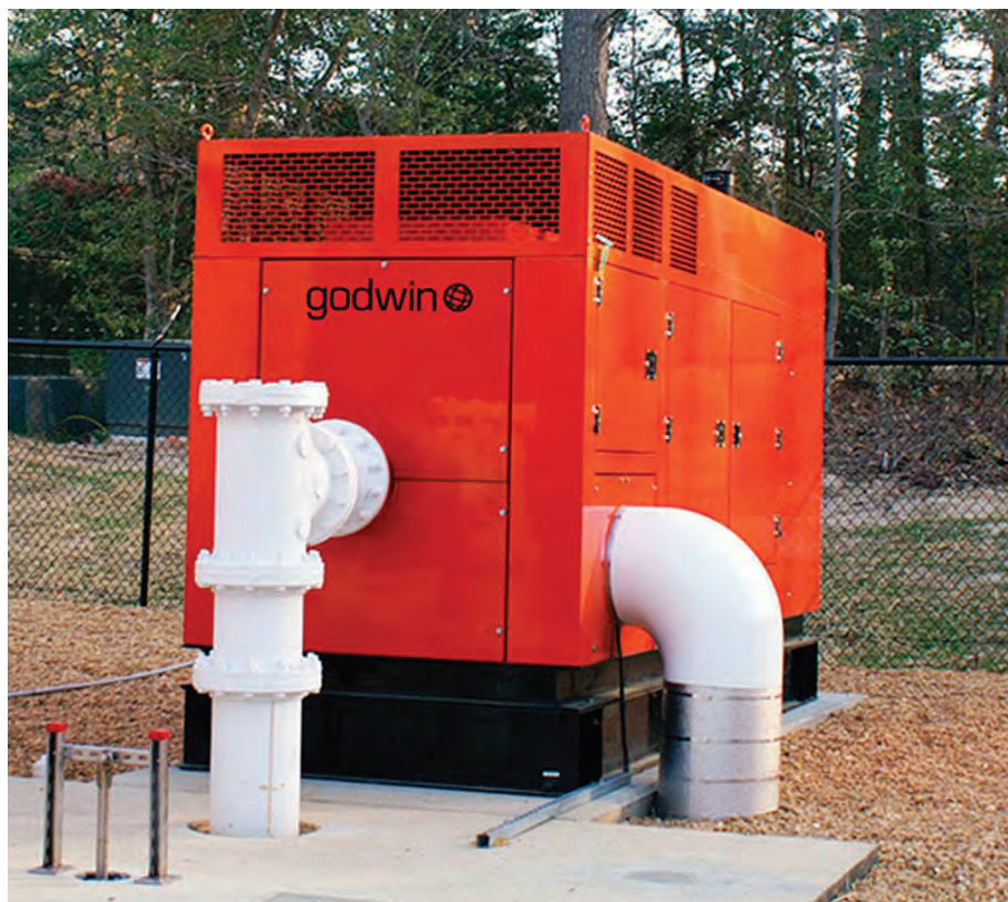
To ensure uninterrupted flow of wastewater, the city has equipped six lift stations with natural gas-powered Godwin Dri-Prime backup pump systems.
