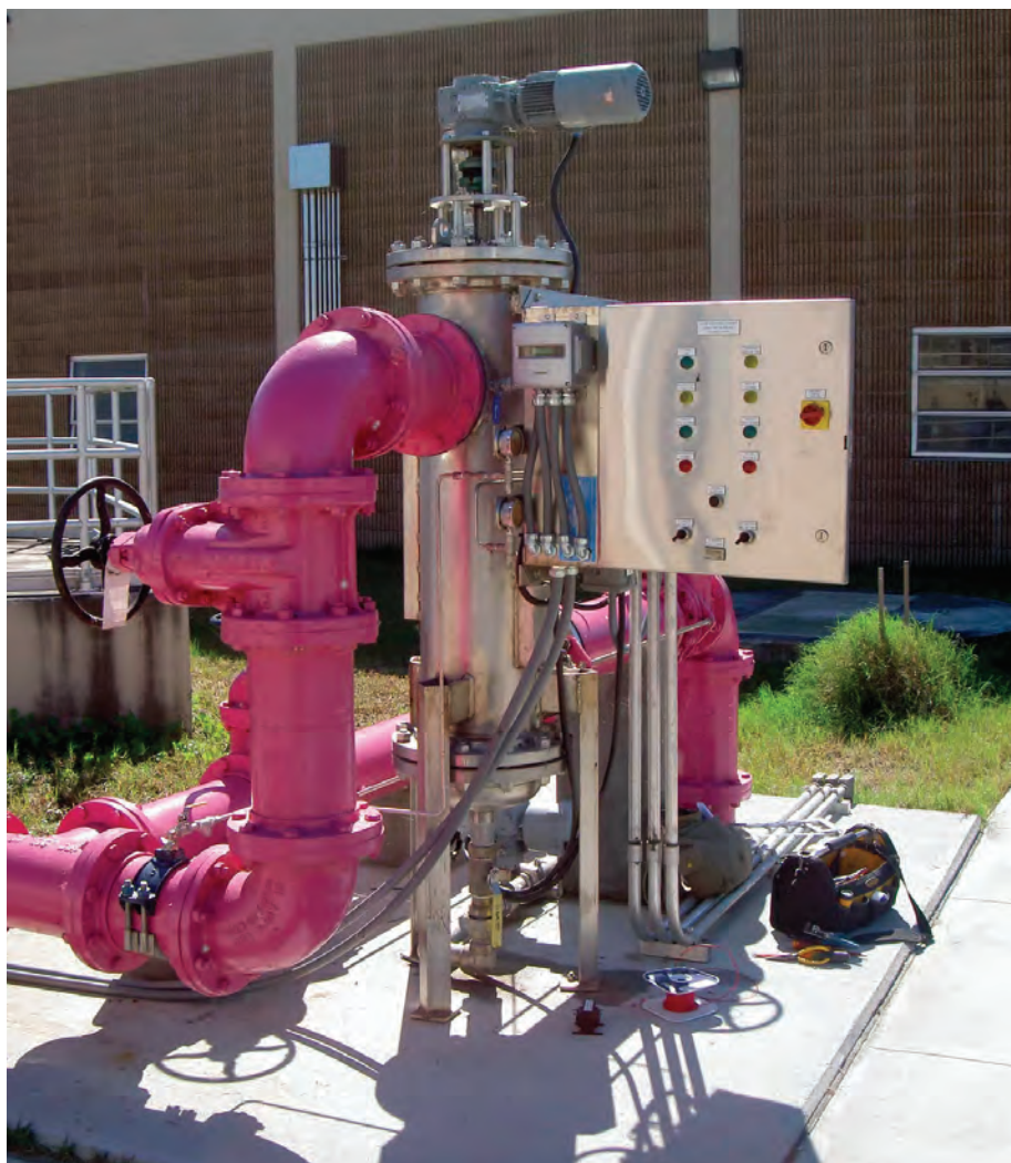
Automated scraper strainers pre-filter water and wastewater to protect fragile membrane systems from damage caused by large, suspended particles, reducing maintenance, and replacement costs.
