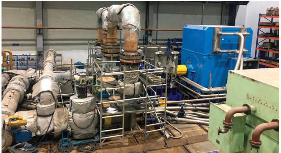
One of the feedwater pumps underwent a thermal shock test as part of the project delivery.
