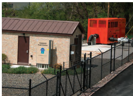
The Fairwood Pump Station is one of six pump stations to be equipped with Godwin Dri-Prime Backup pump units.
