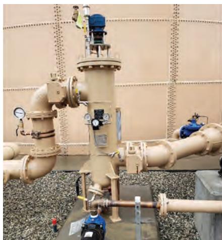
Automatic self-cleaning scraper strainers are increasingly popular because they are affordable, require very minimal maintenance or attention, and can remove solids down to 75 microns.
