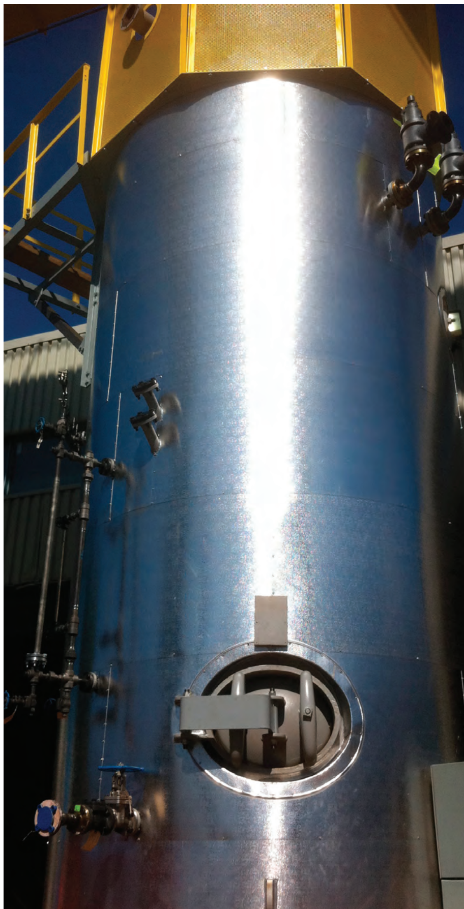
Acme Boilers CEJS high voltage electrode steam boiler.
