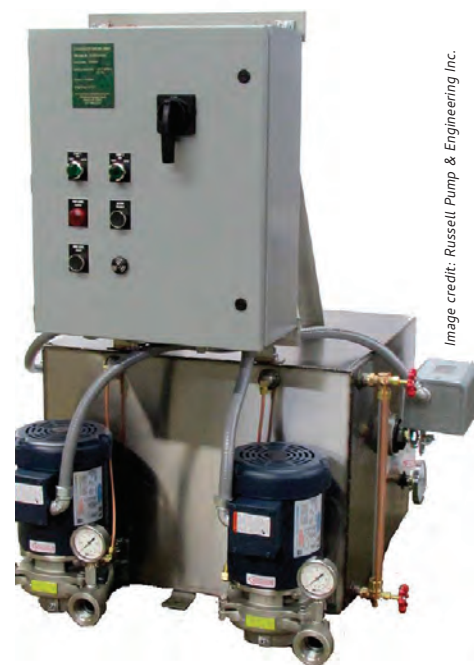
Figure 2: Duplex stainless steel electric condensate pump package
