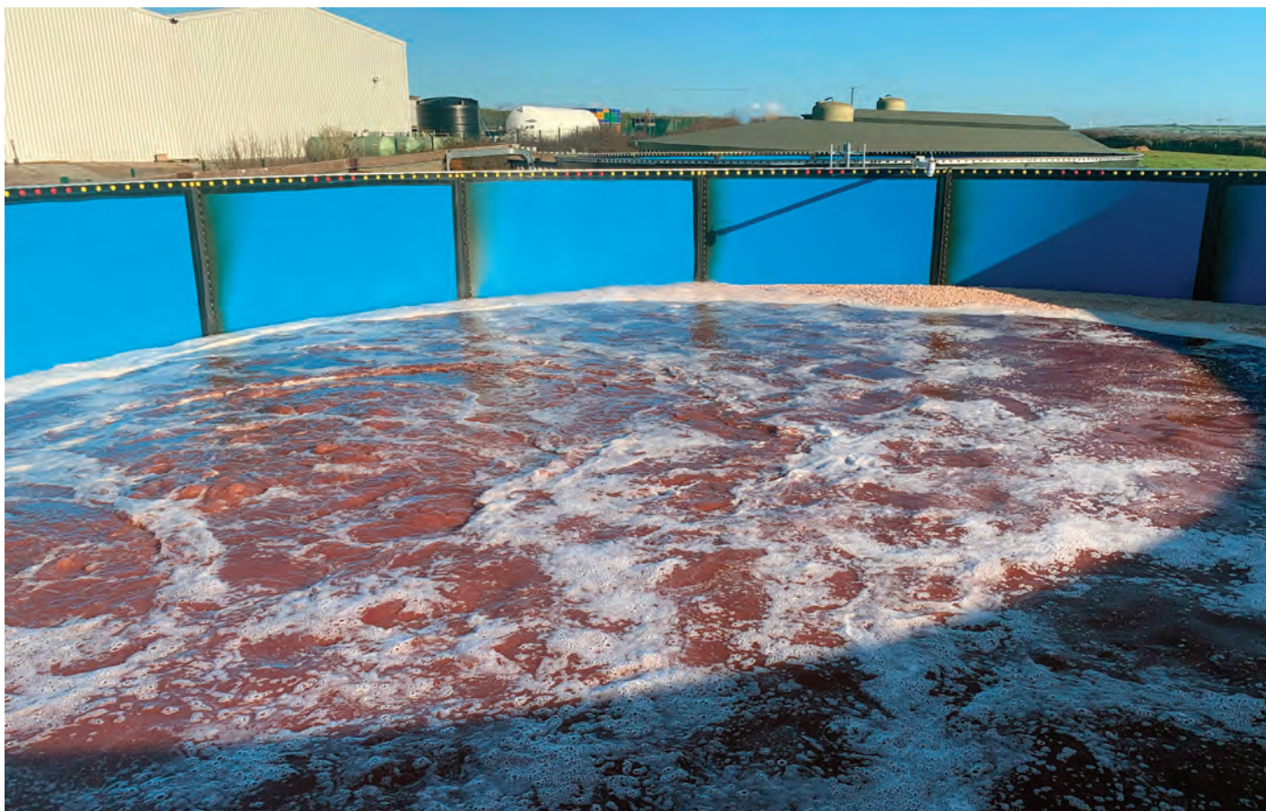
Landia's AirJet (introduced by W.A Cooke & Sons' Watermark Projects Division) aerates a balance tank at a poultry producer in Wales.
