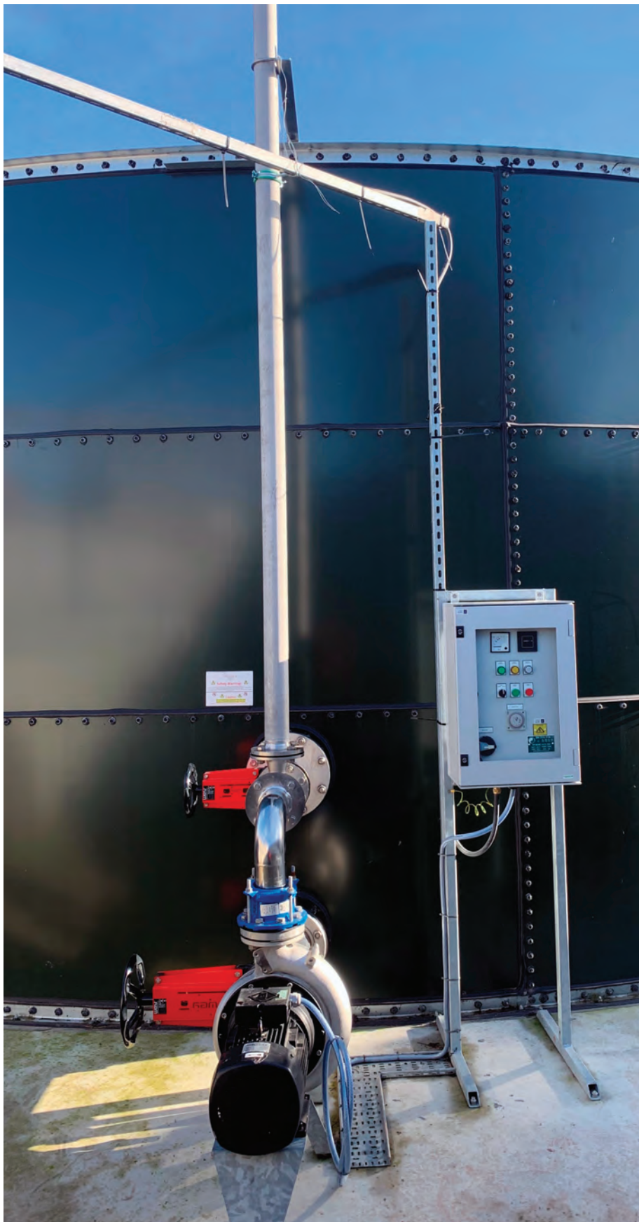
Landia's externally-mounted AirJet, which keeps the balance tank at a poultry producer aerated, ensuring that solids are kept in suspension.
