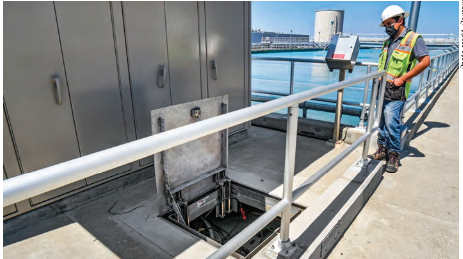
The project included the installation of ten stainless steel floor doors manufactured by BILCO.
