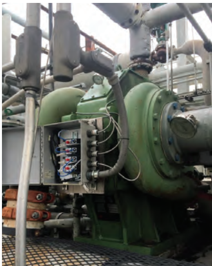
Figure 2: One typical application of a centrifugal air compressor.
