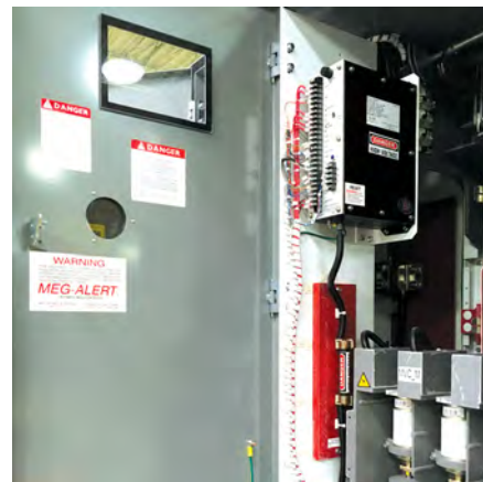
Model GP5000-MU-AS-D1 Motorguard installed in MV MCC.
