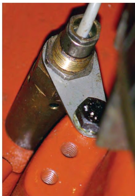
Figure 5: Float switch sensor.
