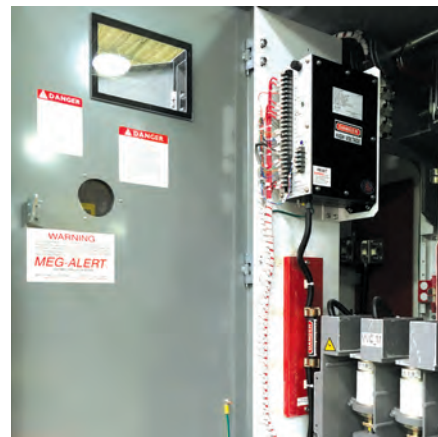
Model GP5000-MU-AS-D1 Motorguard installed in MV MCC.
