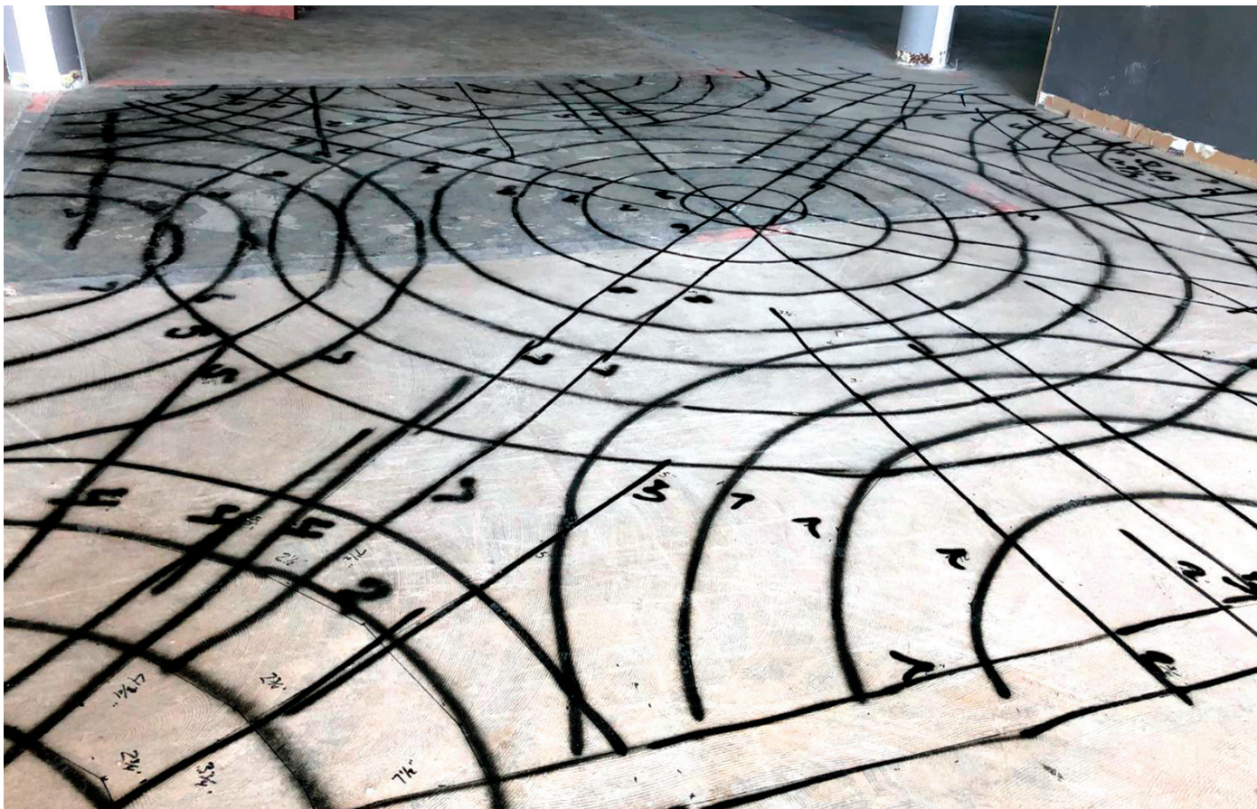
Mark-out of the location and depth of complex circumferential reinforcement design.
