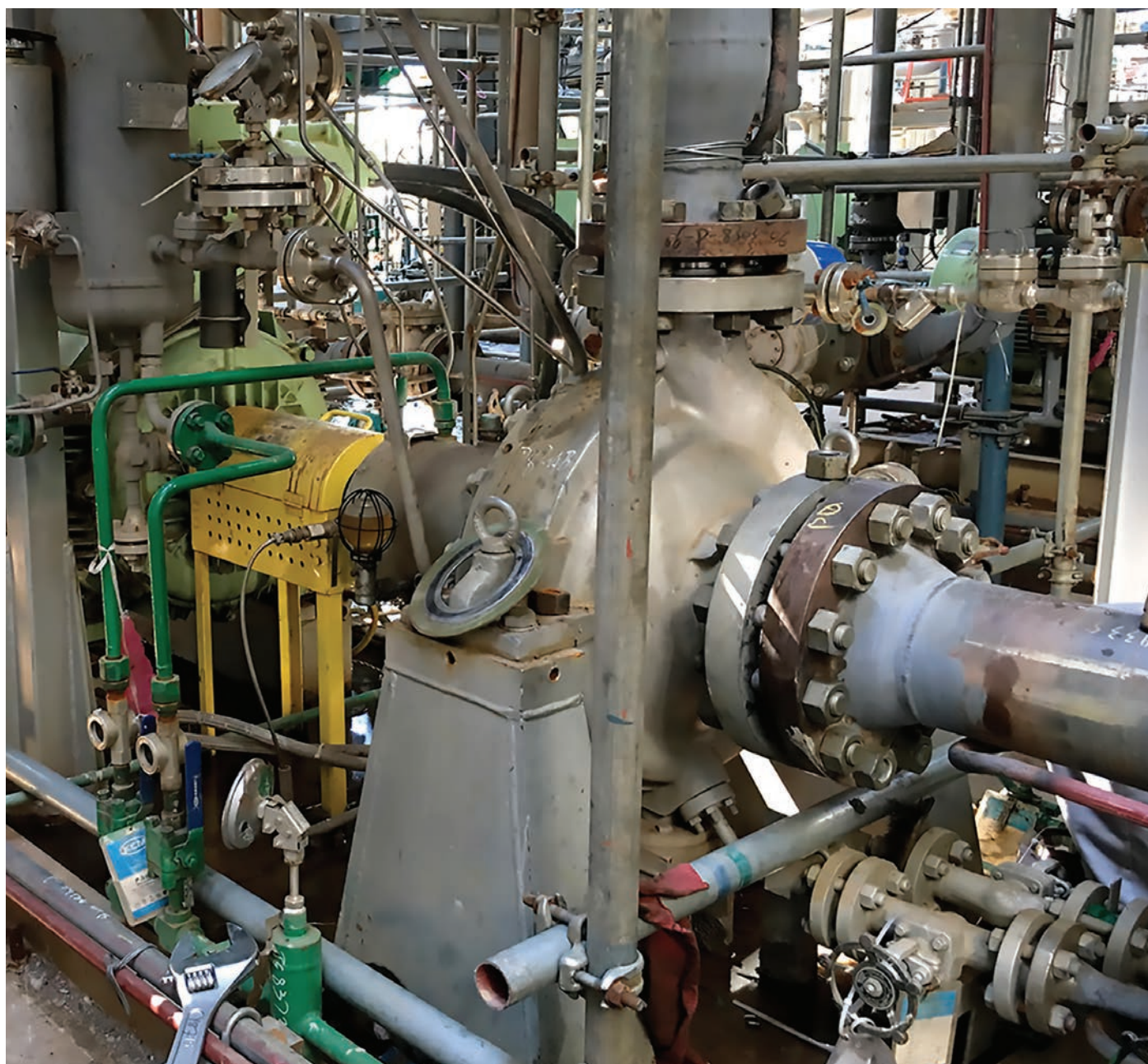
Top: The coke crusher rotor for the large solids abrasive service. Bottom: ZF pump with the coke crusher for the large solids abrasive service.
