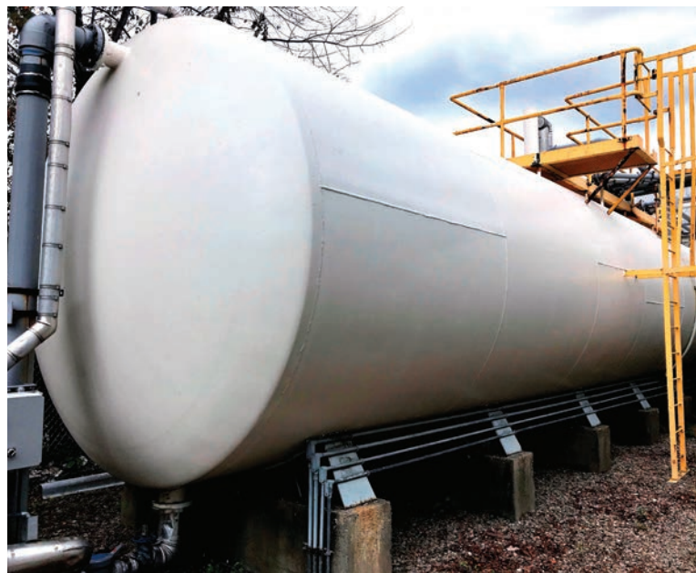
NanoPrime reacts with iron and iron oxide (rust) to form iron phosphate, creating a Nano bond with both metallic and painted surfaces.
