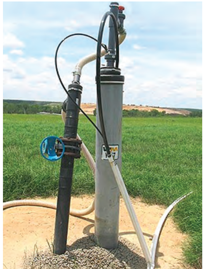
Opposite page: QED AutoPump® models are available to pump fluids up to 250 degrees Fahrenheit (121 degrees Celsius). Top: With QED AutoPumps, the landfill can generate enough energy to power 4,000 homes. Bottom: Waste Management's Springhill Regional Landfill uses QED AutoPumps to dewater gas wells in corrosive, high temperature conditions.
