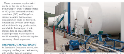
As part of its process, OLVEA Group optimizes storage tanks to ensure oil purity in processing of its vegetable oils and its fish oils.
